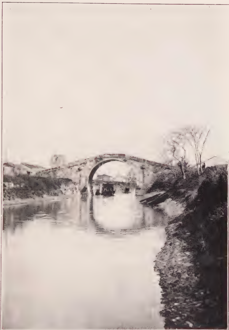
At Tientsin is the northern terminus of the Grand Canal, which extends southward for nearly one thousand miles. In building not only this waterway but also the hundreds of high-arched bridges that cross it, the Chinese have proved themselves first-class engineers.
